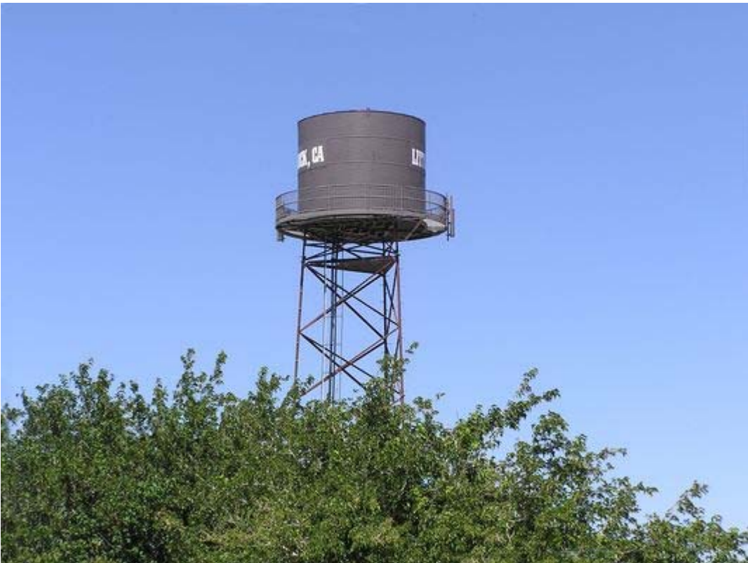
Figure 13: Faux water tank wireless site in Littlerock, California
