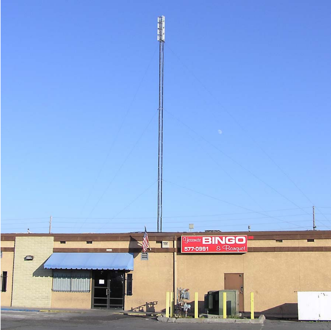
Figure 2: Guyed roof-top wireless tower site in Modesto, California.
