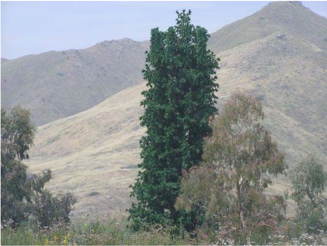
Figure 7: Superior Monopine wireless site in Lake Elsinore, California.
