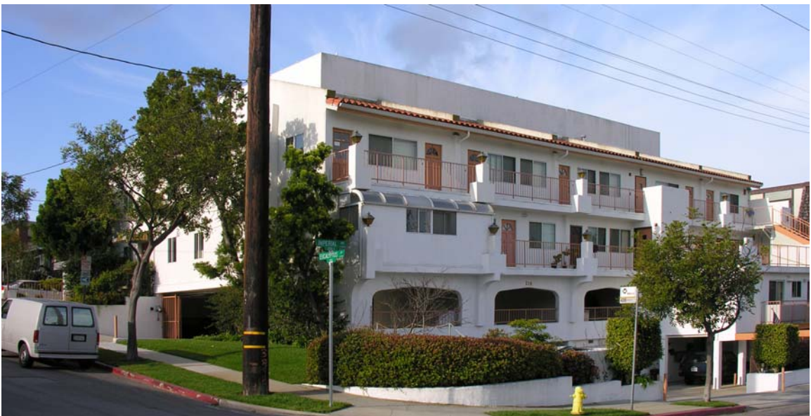
Figure 10: Wireless site hidden behind roof parapet in El Segundo, California.
