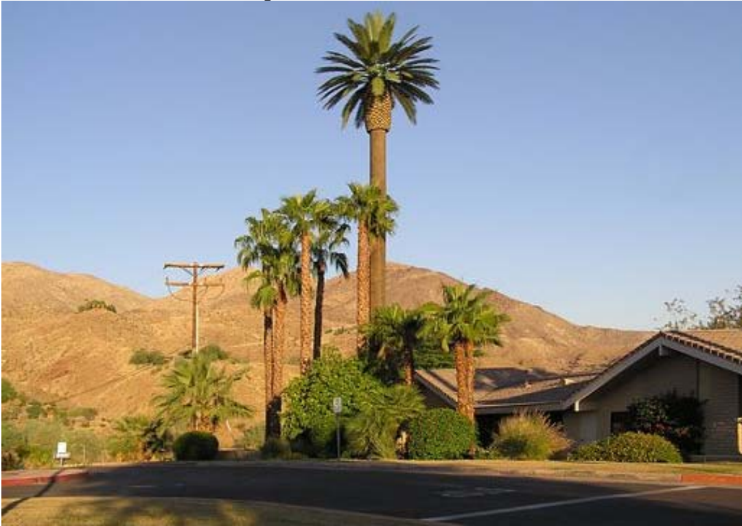
Figure 8: Superior Monopalm wireless site in Palm Desert, California.
