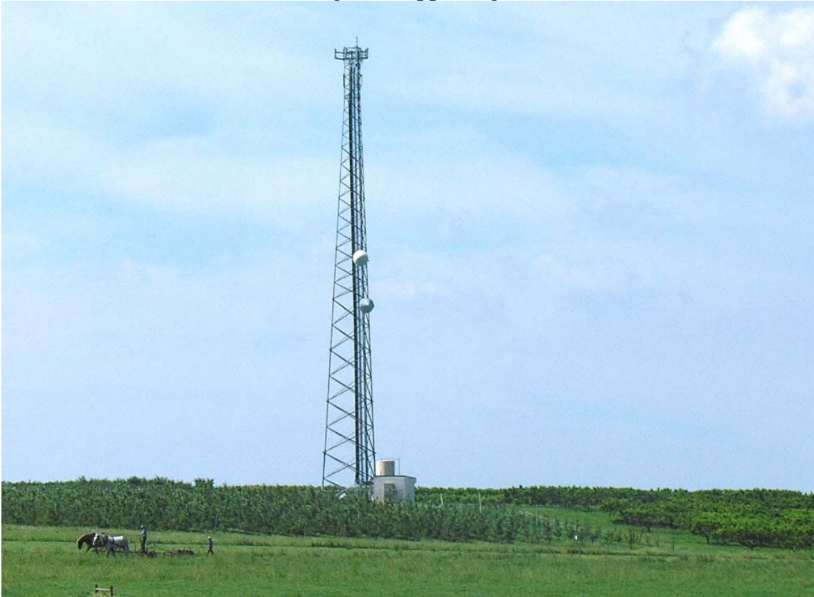
Figure 1: Self supporting wireless tower site in Bird-in-Hand, Pennsylvania. 18
