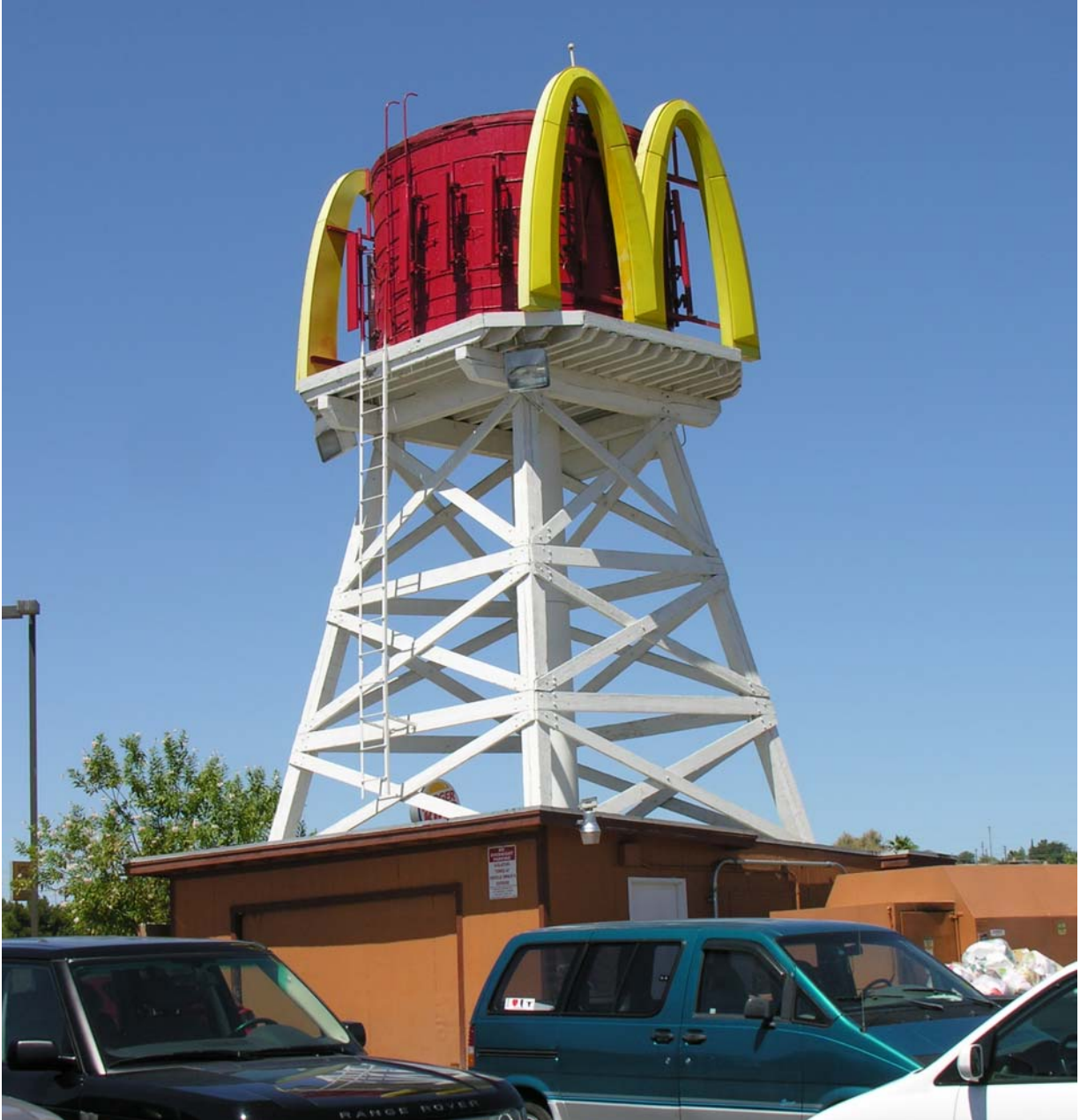
Figure 11: Faux water tank/advertising sign wireless site in Barstow, California
