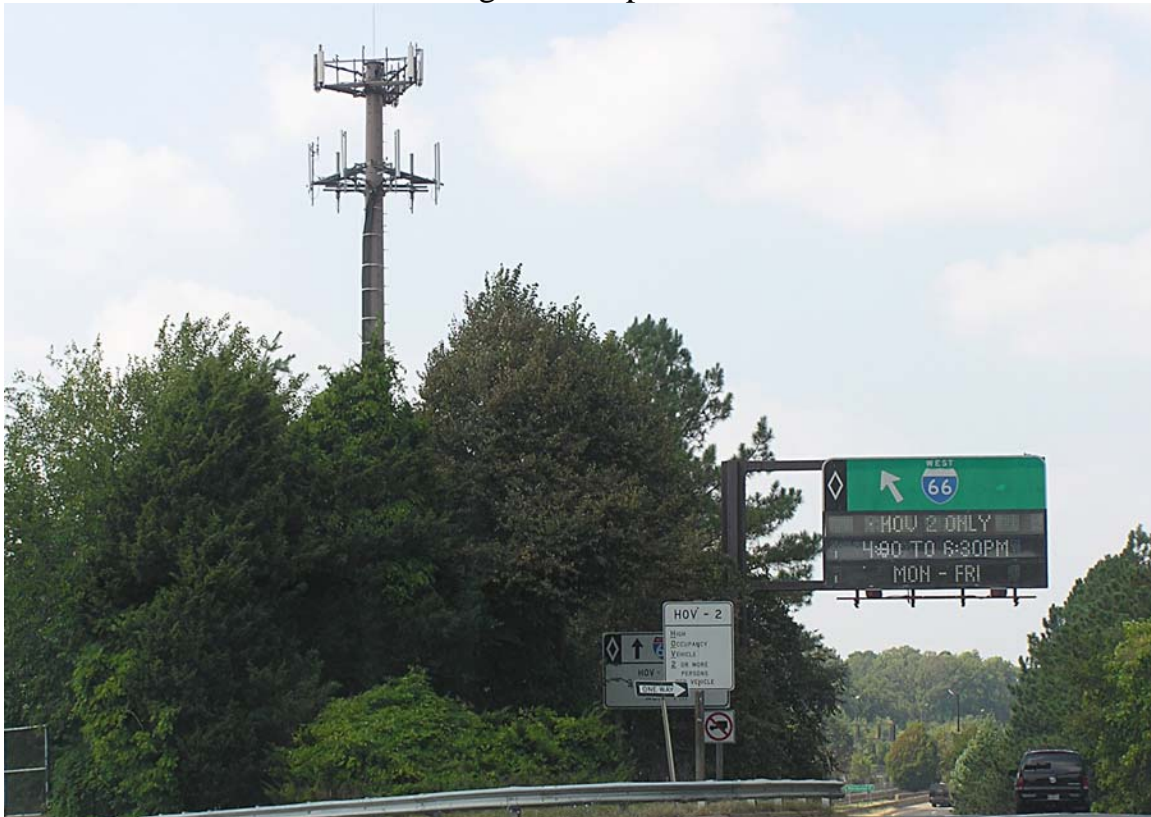
Figure 3: Uncamouflaged Monopole wireless site in Fairfax, Virginia.
