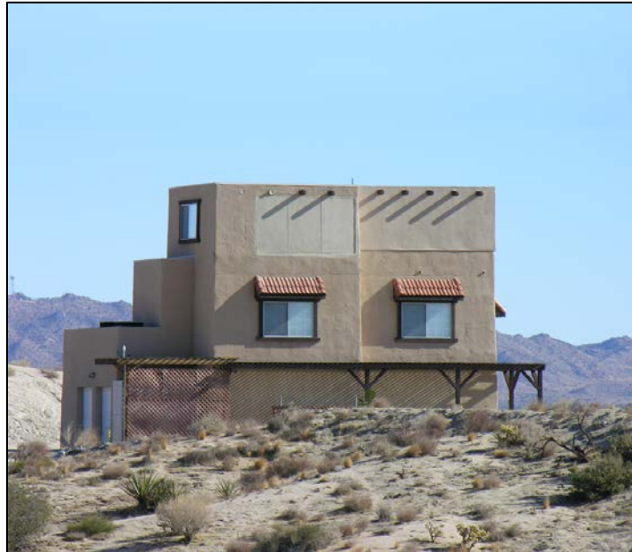
FIGURE 4: Actual photograph of an unmanned camouflaged wireless site in Yucca Valley, California. (Source: Telecom Law Firm, P.C.)
