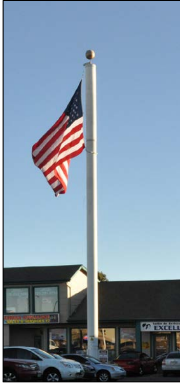
FIGURE 2: Camouflaged site in Denver, Colorado. (Source: Telecom Law Firm, P.C.)
